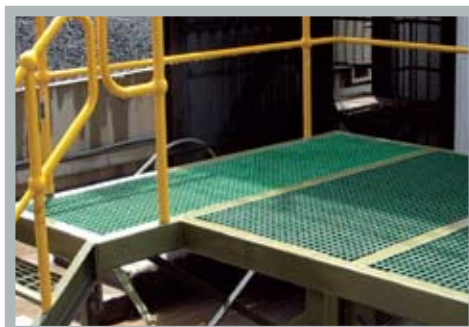
Concrete batching plant, Busselton, WA
